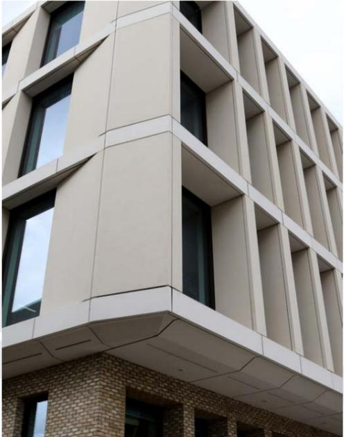
**The external cladding comprises of 692 plain and 459 Brick faced GRC panels, which combined total approximately 4000sq.m of surface area.**
